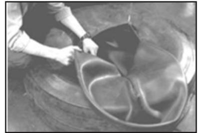
3. Position the tire bead area (where the wires cross the bead) so the cable is lined up with the curing tube stem and stem slot in the rim.
