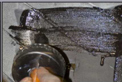
Apply Cement to Repair Area
