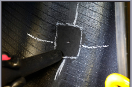
Vacuum the Repair Area
